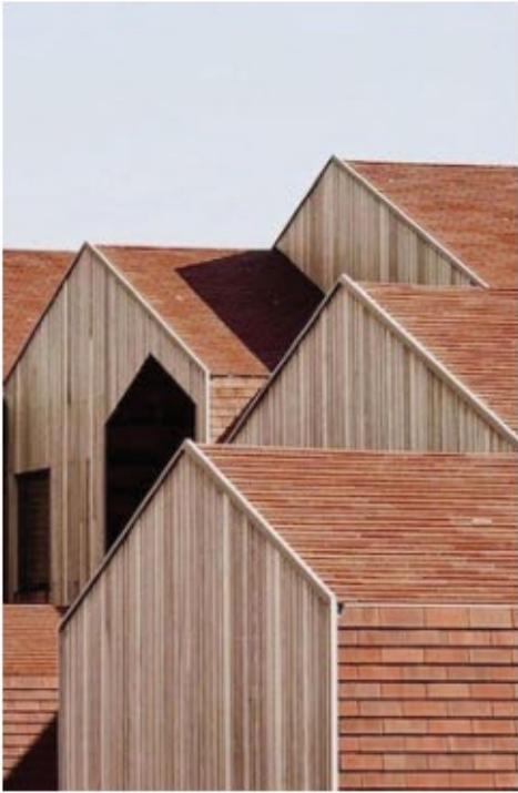
Precedents for contemporary hung tile projects. Clay tiles are used for roofs in the area and the warm palette would harmonise with buff brickwork proposed for the ground floor and the gable.
